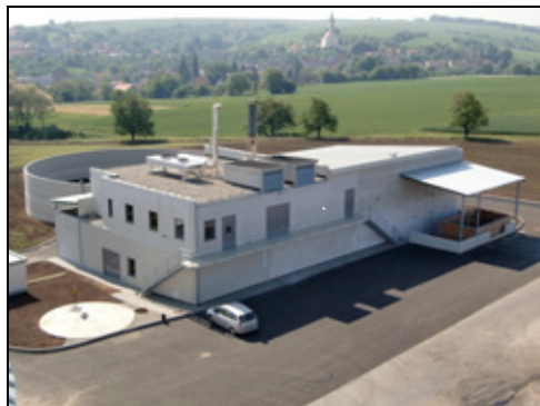
Fig.1. Biogas plant of Enserv Rys. 2 Biogazownia Enserv
