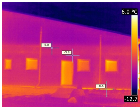
Figure 4. West façade of piggyery (part 1)
